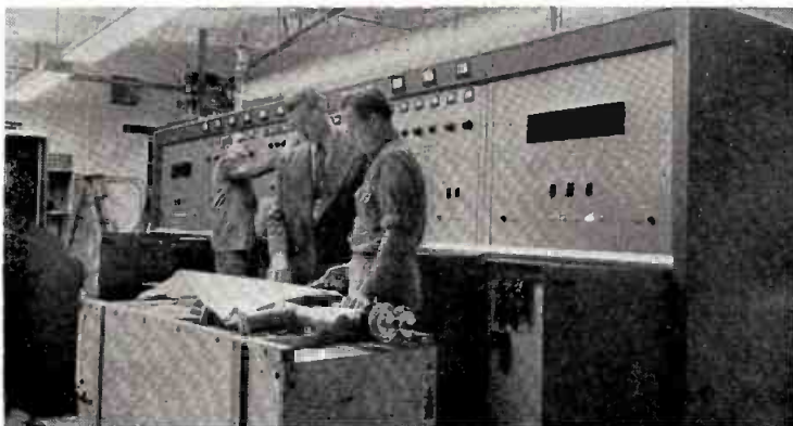
G-E field engineers Stone, Bias and Duncan (l. to r.) work on the installation of the first 12-kw transmitter built by G.E. for WHUM-TV.
